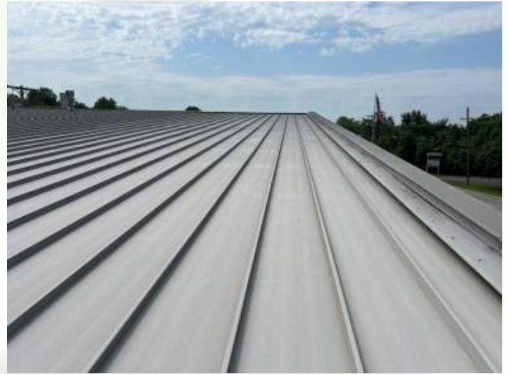
West perimeter South view
