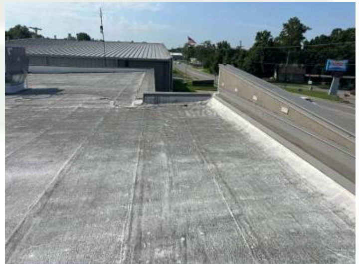
West perimeter edge South view
