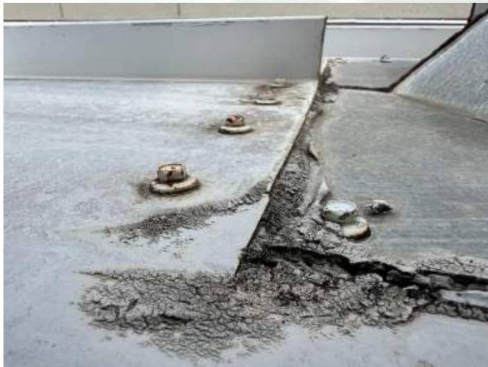
Close-up of the sealant and fasteners at the roof penetration
