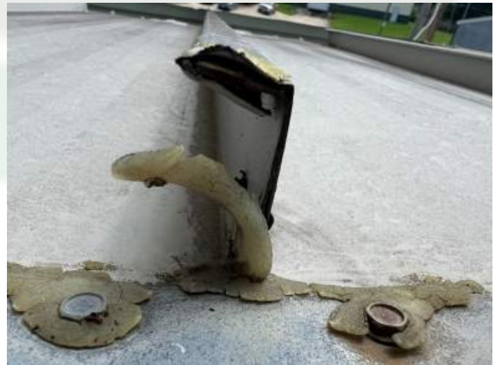
End of the standing seam at the roof penetration
