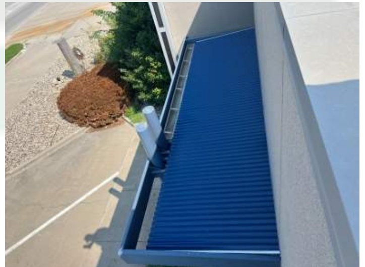
Roof surface North view
