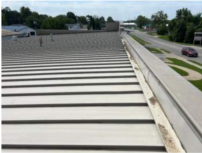
West perimeter edge South view
