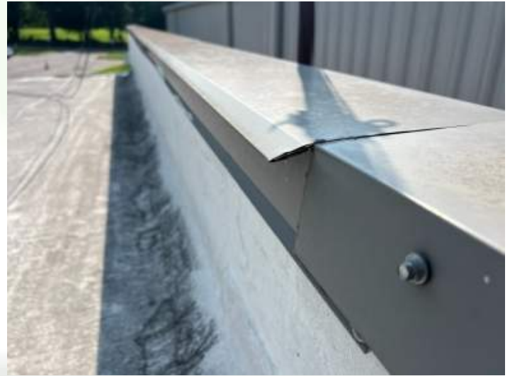
South perimeter edge East view
