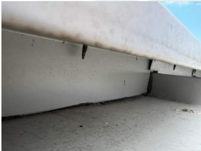
Closures shown beneath the metal fascia metal on the South perimeter
