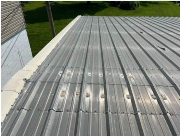
North perimeter edge East view
