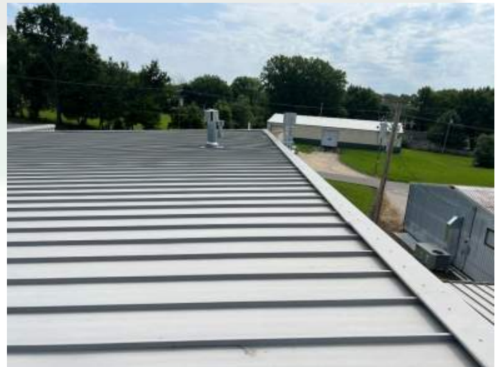
South perimeter East view
