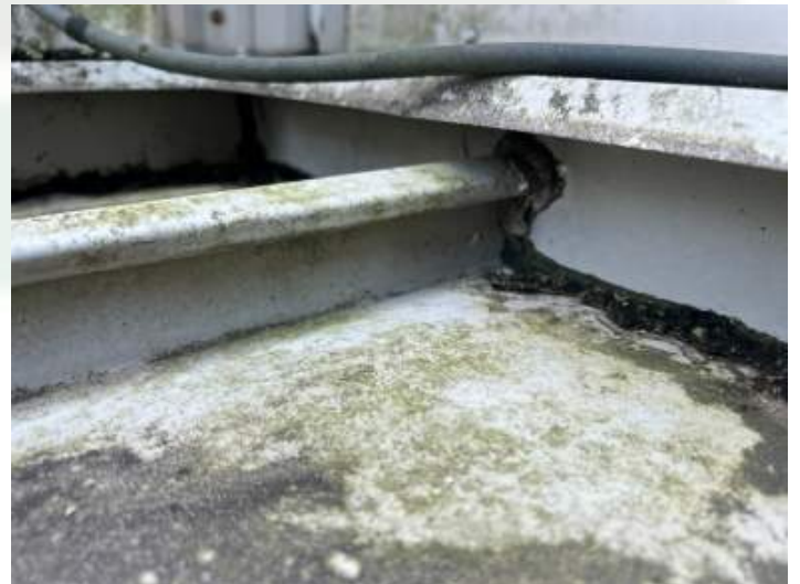
West perimeter with end closures sealed
