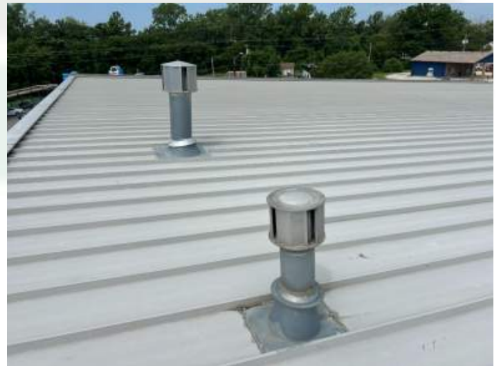
Multiple penetrations are recommended to be sealed
