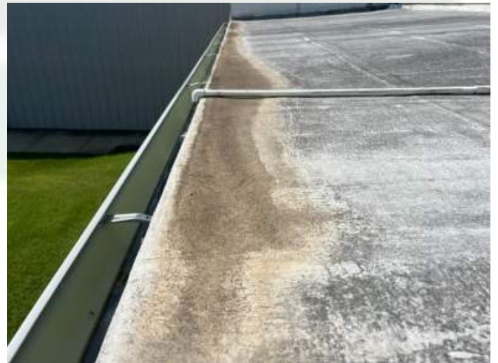
Lower section East perimeter gutter edge
