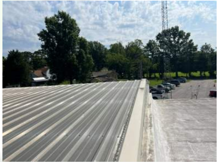
South perimeter edge East view
