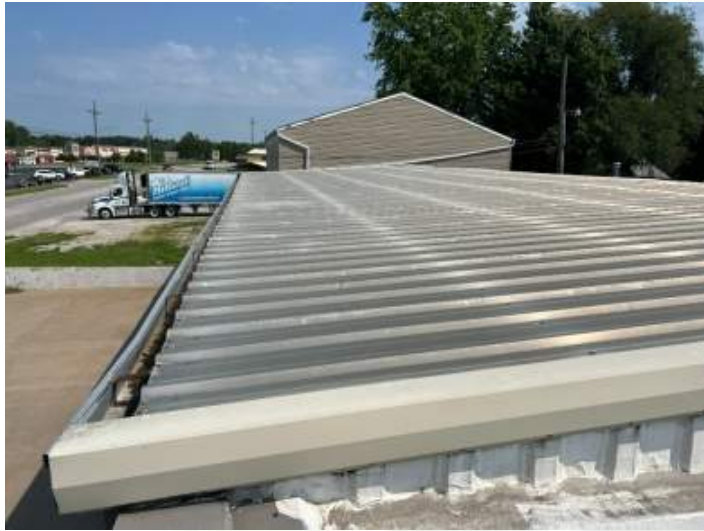
West perimeter edge North view
