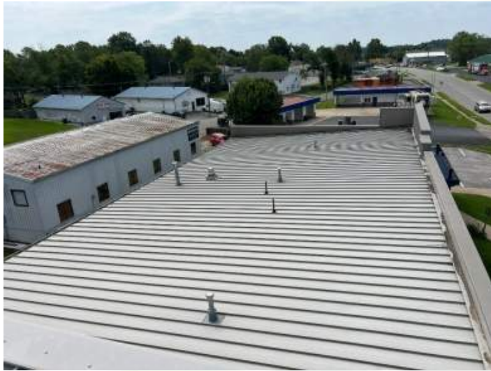
Roof surface South view
