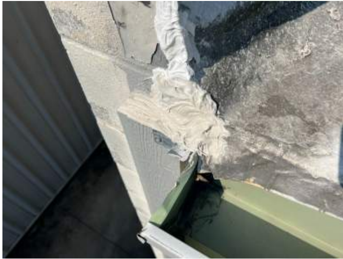
Patch repair at corner roof edge
