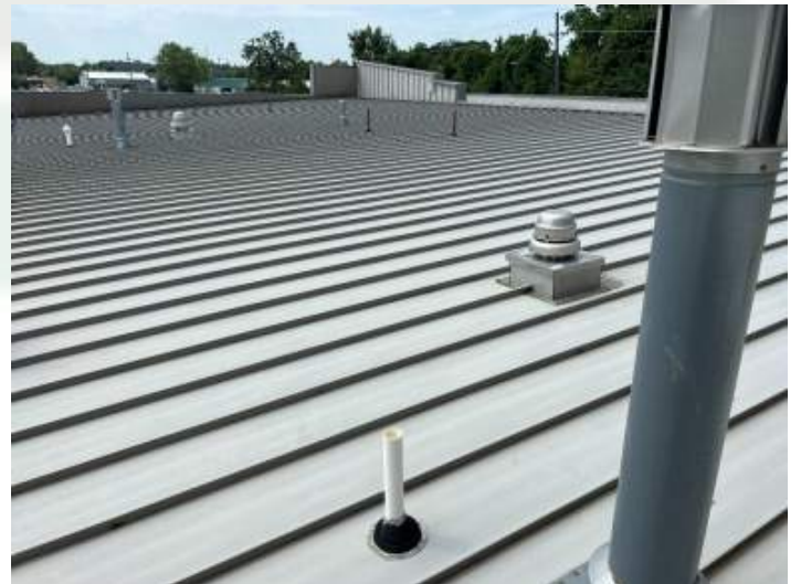
Roof surface South view
