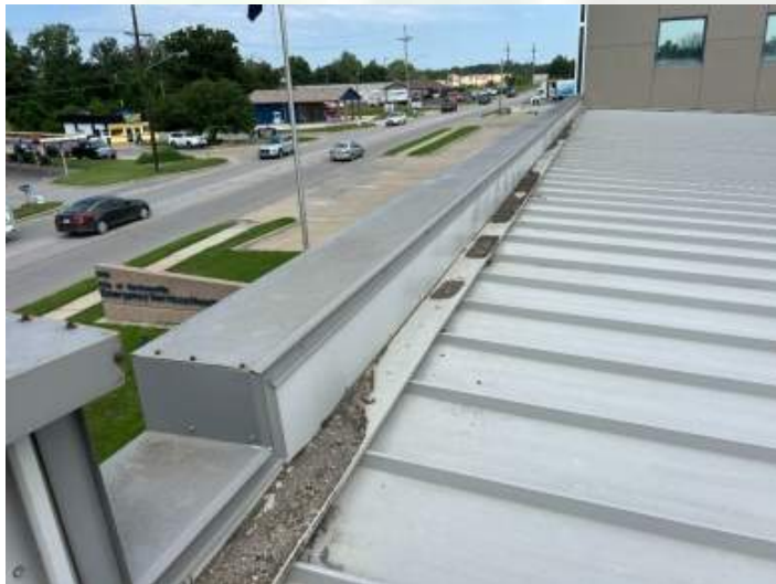
West perimeter edge North view
