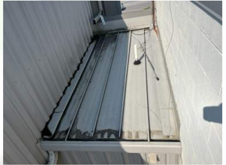
Roof surface West view
