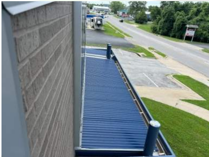
Roof surface South view
