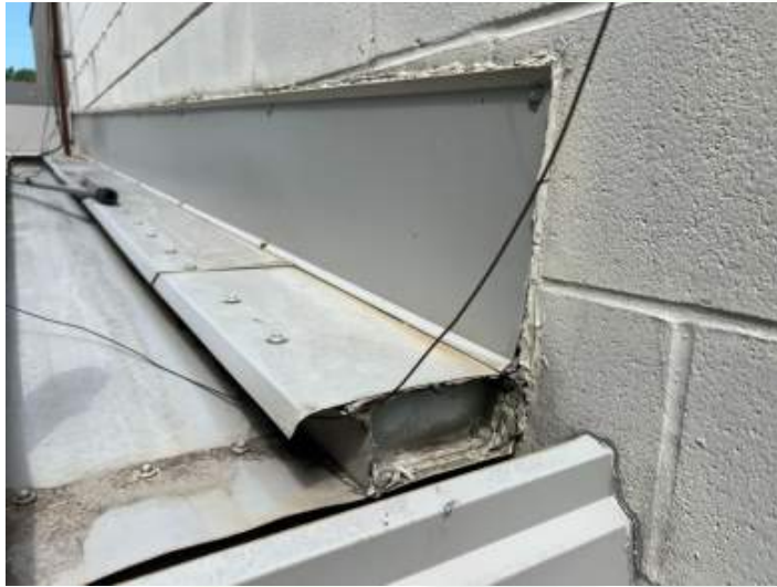
North perimeter wall flashing West view
