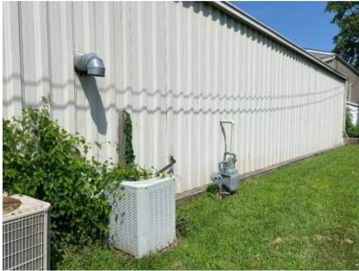
East wall with penetrations
