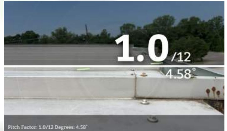
1" by 12" pitch or slope to gutter edge
