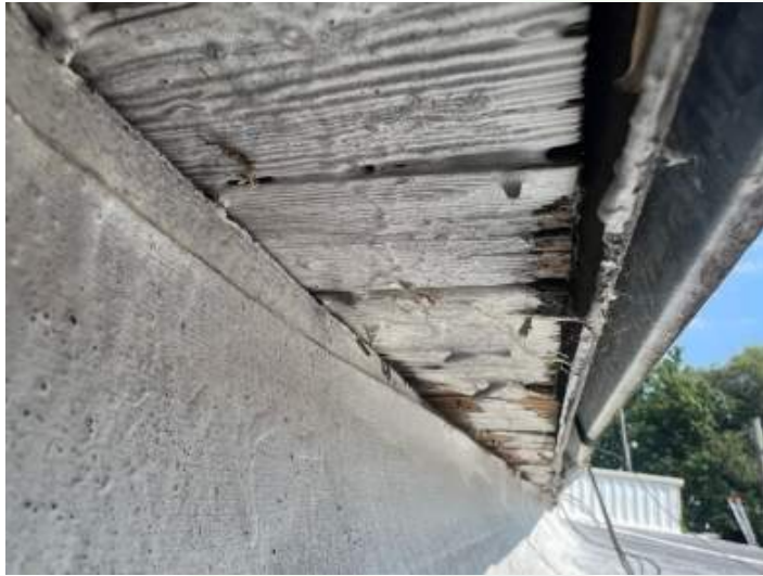
Upper roof section beneath the overhang
