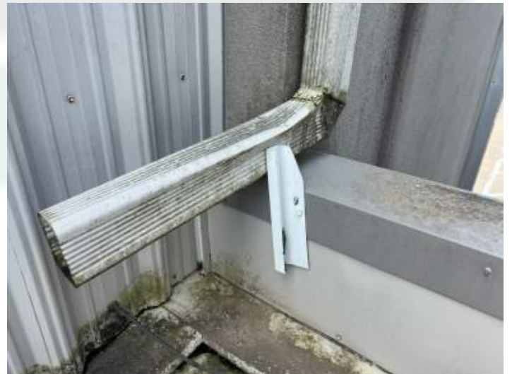
Secured downspout with a metal brace
