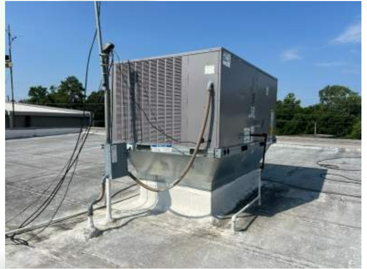
Mechanical equipment & multiple linesets
