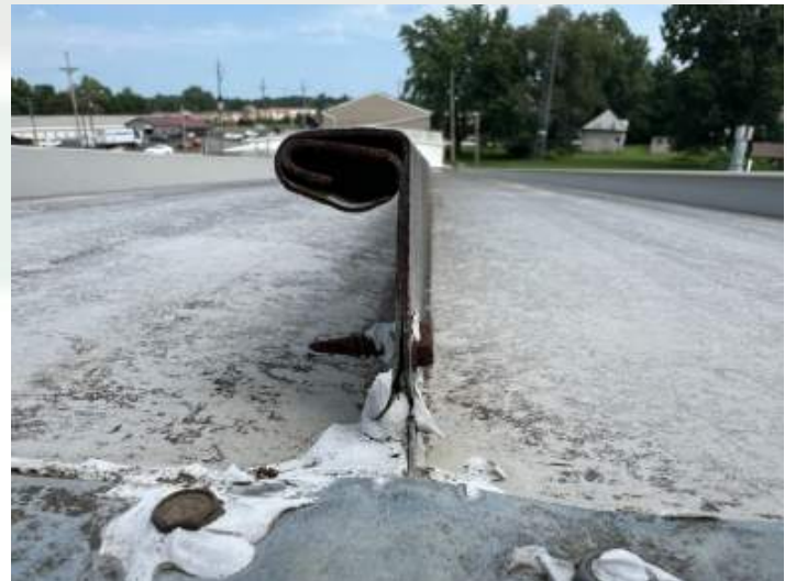
Rib end close-up to show the seam with failing sealant
