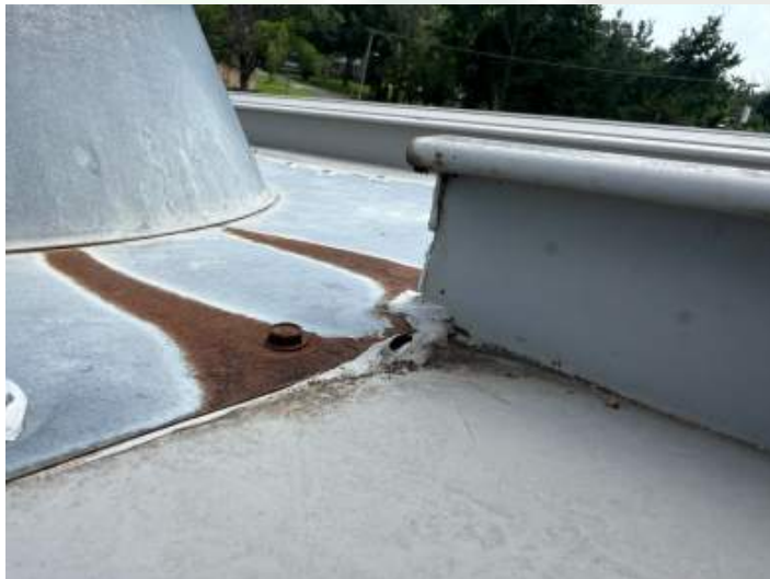
Ribs in standing seam metal were cut to install pipe flashing
