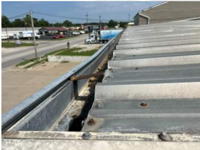
West perimeter gutter edge North view
