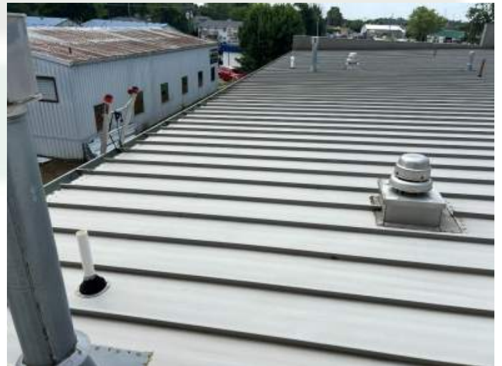
Roof surface South view
