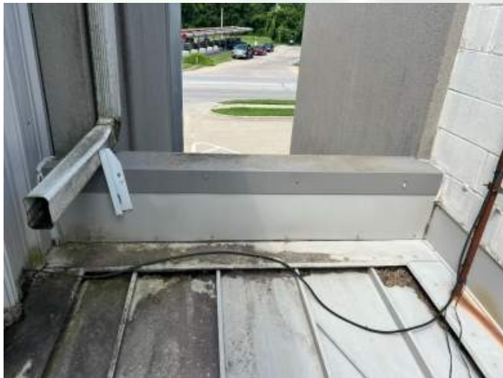
West perimeter edge with downspout draining onto from upper roof section
