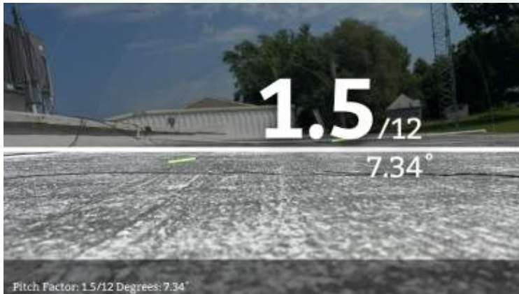
1.5"/12" pitch on the lower roof section with gutter system
