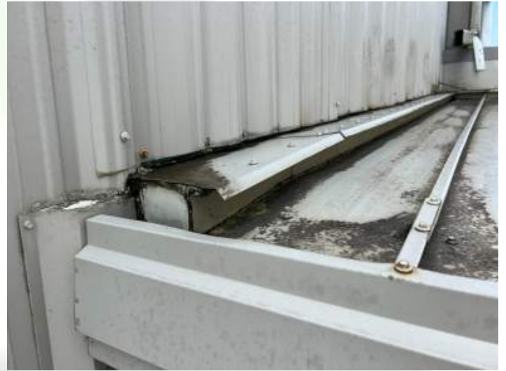
South perimeter wall flashing West view
