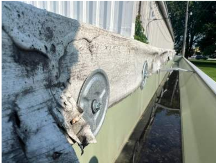
Gutter edge coating and supportive mesh secured with fasteners and plates
