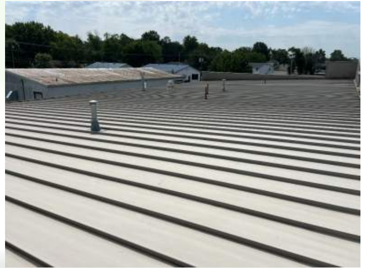
Roof surface view
