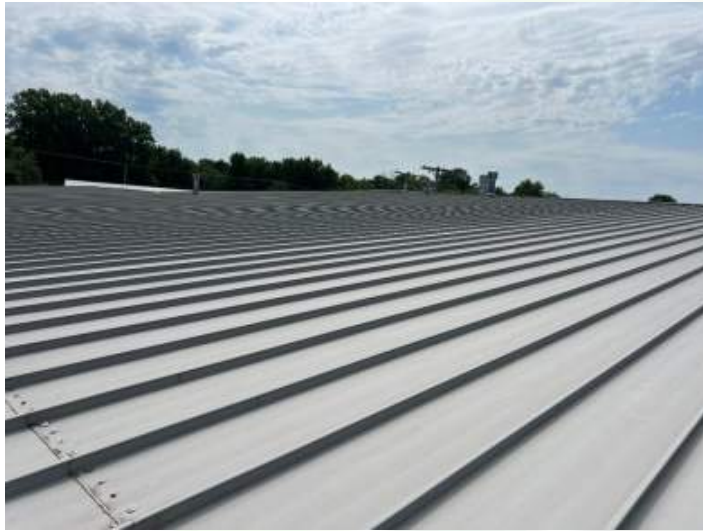
Roof surface view
