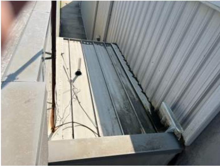
Roof surface East view
