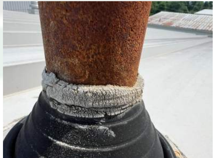
Deteriorated sealant
