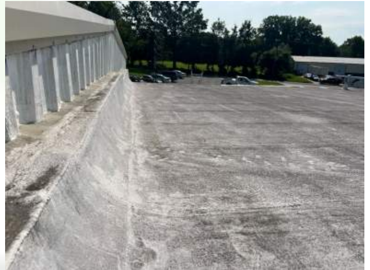
North perimeter tie in to the building wall
