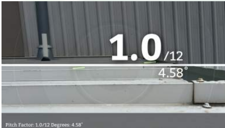
1" by 12" pitch or slope to gutter edge
