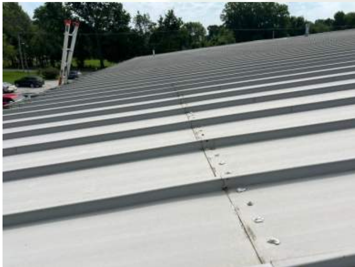
North perimeter East view
