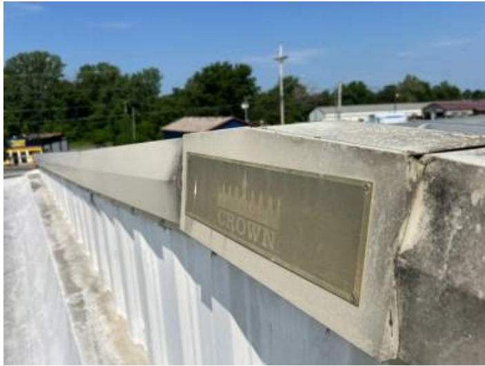
Manufacturer appears to be Crown shown at the ridge end cap
