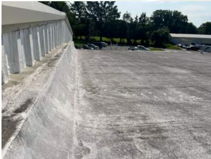
North perimeter edge East view
