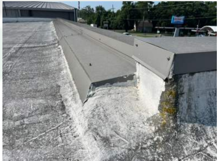
West perimeter edge with coping cap metal and top fasteners
