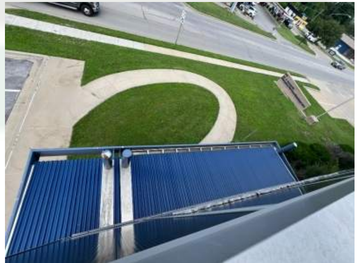
Roof surface view
