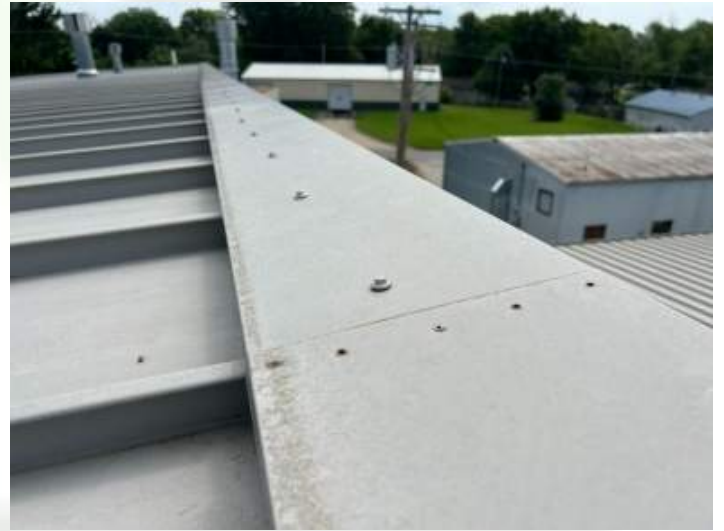
South perimeter edge East view
