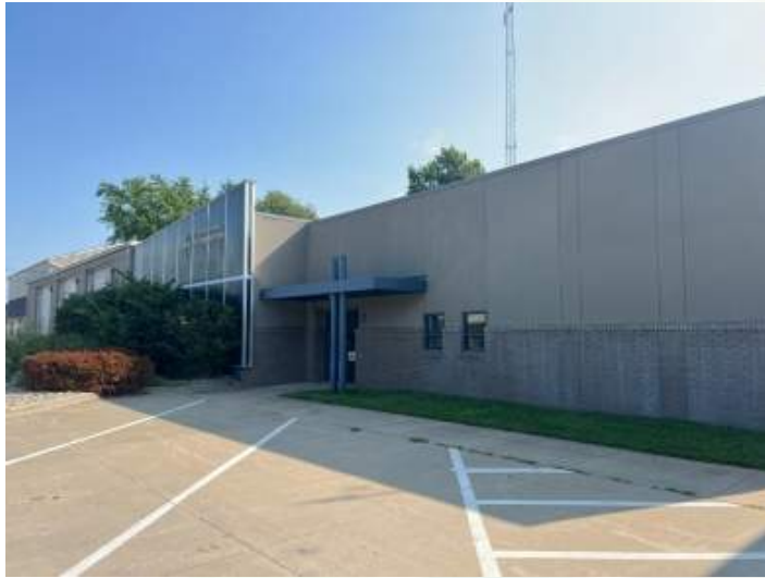
Awning roof North end
