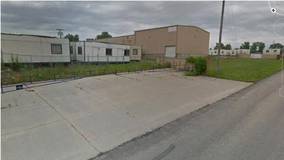
Note: Modular offices from prior tenant have been removed.
