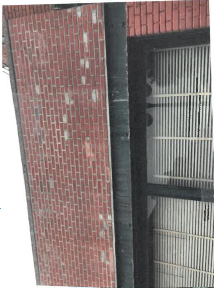
North Panel Facade
