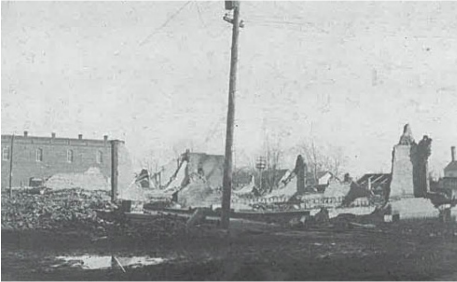
A fire in February 1900 destroyed all the buildings on the south side of the square. The buildings were replaced with new ones by the end of 1902. (image from page 32, Bohl/Atkinson)
