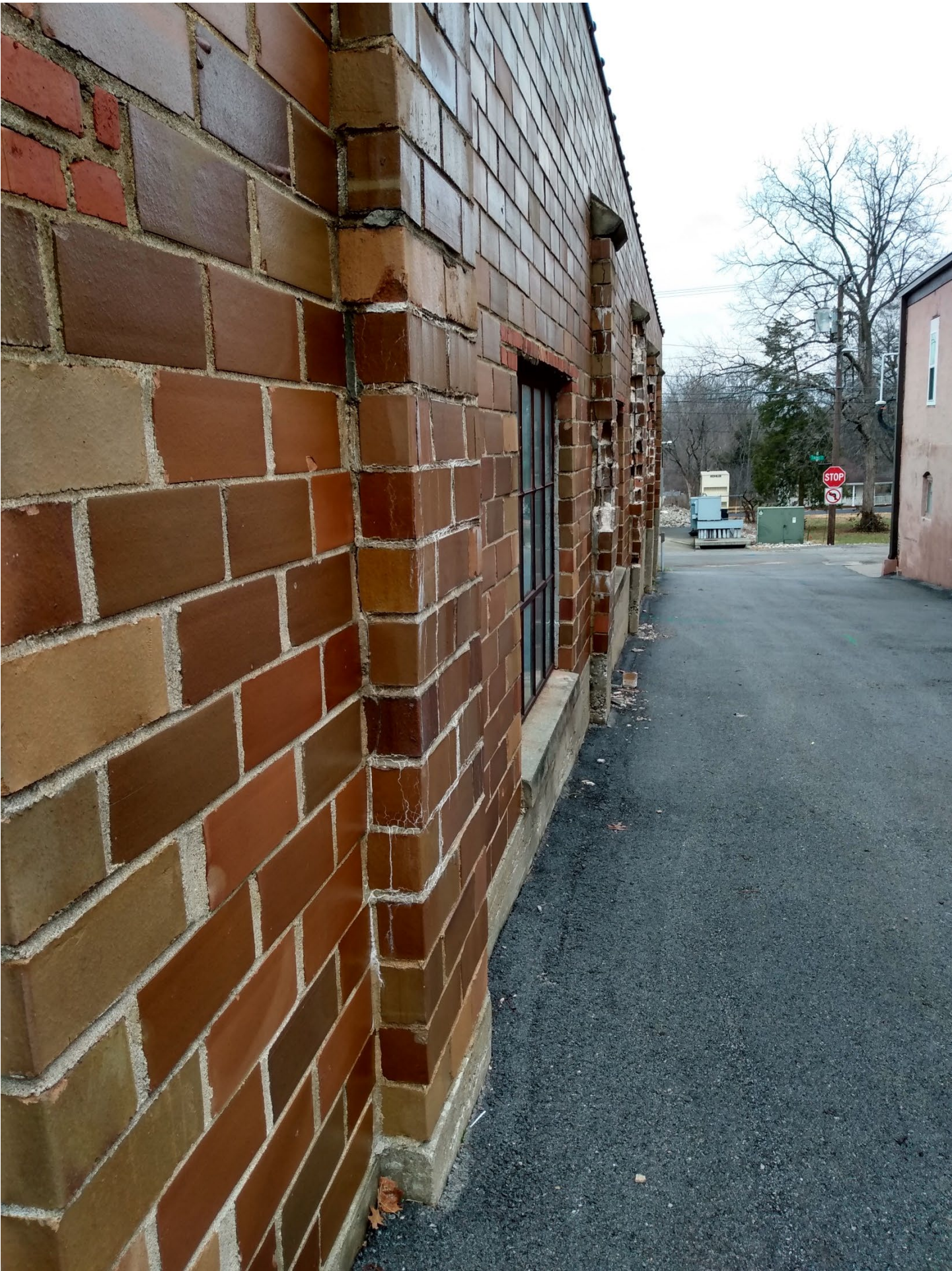
Attachment: Pictures (COA for Partial Demolition at 208 E. Pearl St.)
