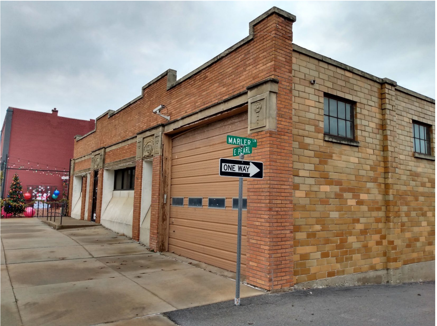
Attachment: Pictures (COA for Partial Demolition at 208 E. Pearl St.)
