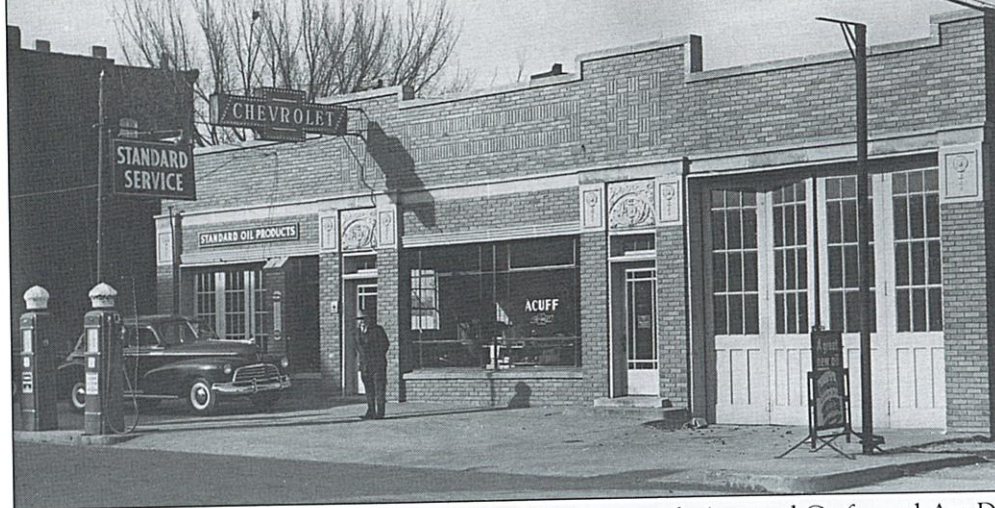
208 EAST PEARL STREET, 1947. This buff-brick building with Arts and Crafts and Art Deco elements was built in the 1920s for the White Motor Company. Herb Acuff owned it from 1959 until 1964, when it became Moore-McLain Chevy/Olds. It housed Need's Body Shop in the early 1970s. It was converted into the Harrisonville Police Station in 1977 and was later used as a community center. (Courtesy of Janet Allbaugh.)
