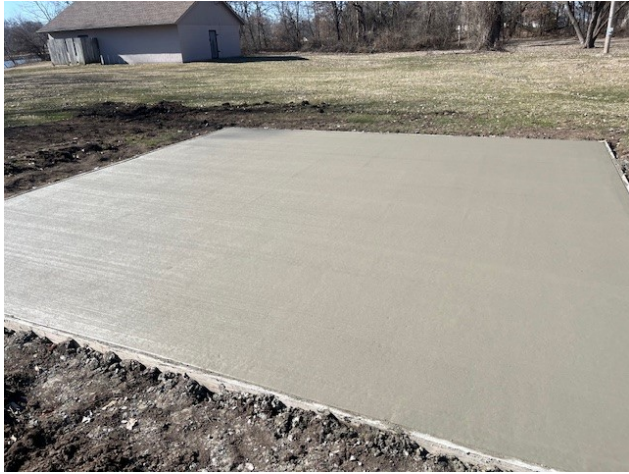
Gaga Ball concrete pad – Camp Reeder
