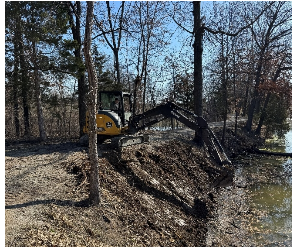
Removed damaged tree from trail
