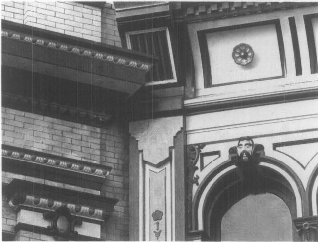
Detail of polychromed cast-iron facade at 23 Petaluma Boulevard, Petaluma, Calif. (1886; O'Connell and Lewis, Architectural Iron Work , San Francisco). Photo: Don Meacham.
