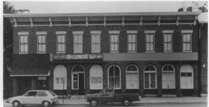
Figure 5. In some cases, as in the storefront on the extreme left, it is a simple matter to determine original appearance by looking at neighboring storefronts. Removal of the board and batten fasciaboard, pent roof, and "colonial" style door, all of which could be undertaken at minimal cost, would restore the original proportions and lines of the building. Photo: Day Johnston
