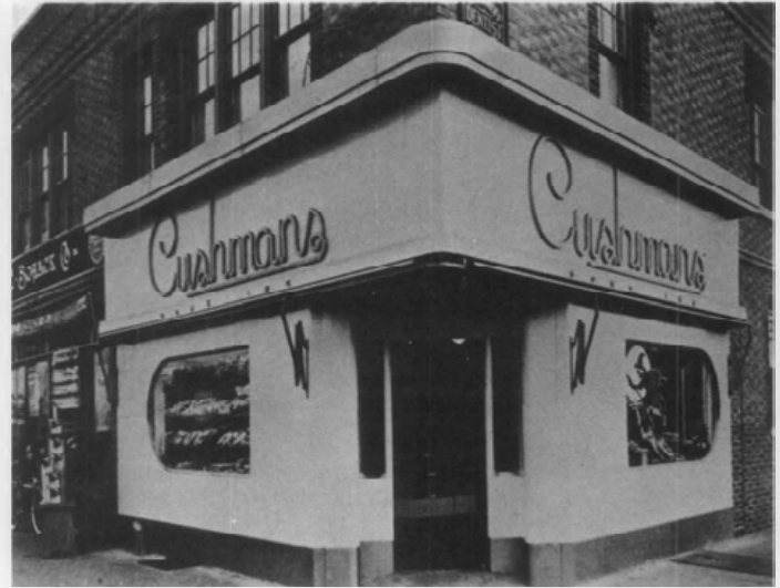
Figure 4. This storefront in New York City designed by Raymond Loewy typifies the streamlined look of the 1930's. Added to an earlier building, the front utilizes glass, stainless steel and neon to make a modern statement. This is a good example of a later storefront which has acquired significance and should be retained in any rehabilitation.
